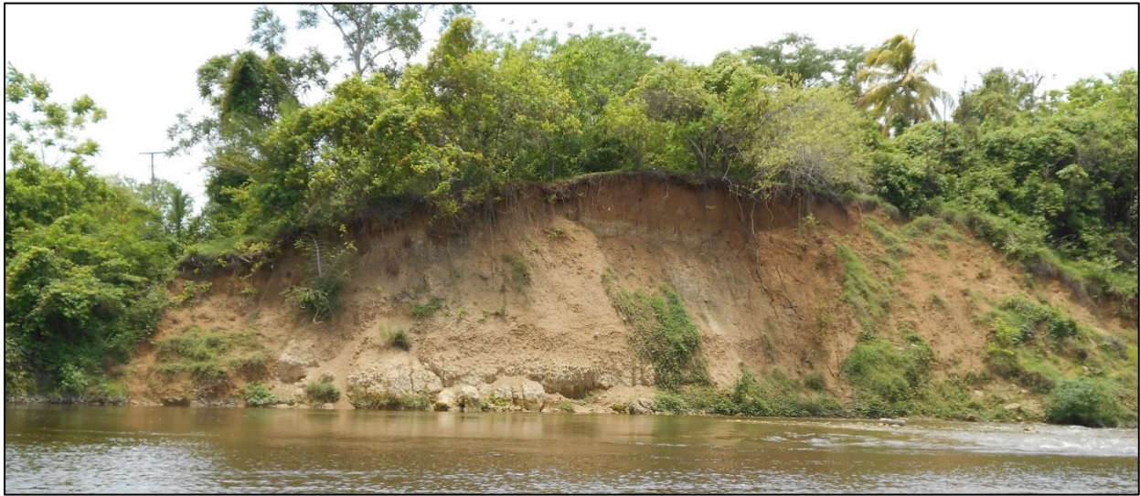
Figure 5.2. Overview of the cutbank containing KS001 in the upper stratum of the cutbank. The lowest stratum with large peds in the center of the image is the paleosol reported to have contained the sloth bone noted above.
