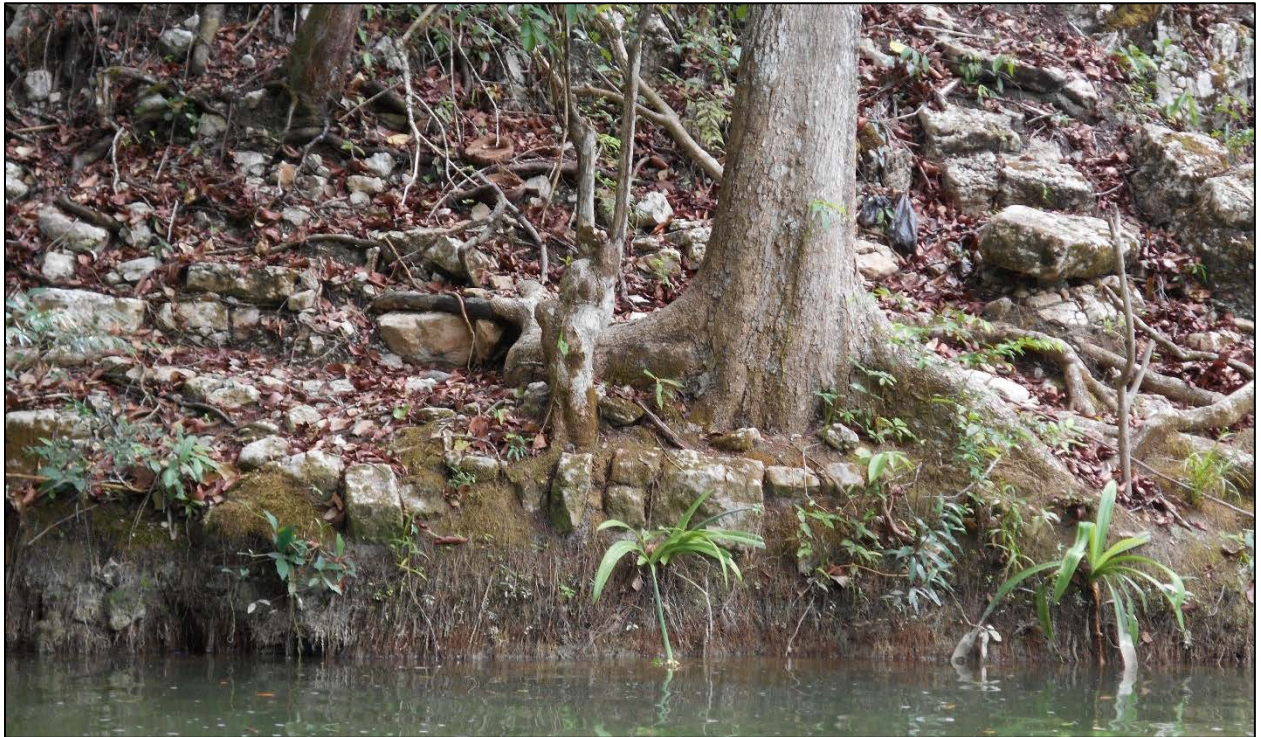
Figure 5.5. Close-up of the eroding structural blocks at the base of KS002. Note what may be the lowest building blocks on a cleared surface near the water level.
